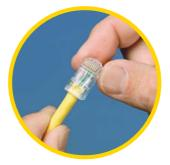
**STEP 7** Slide assembly into plug body.
